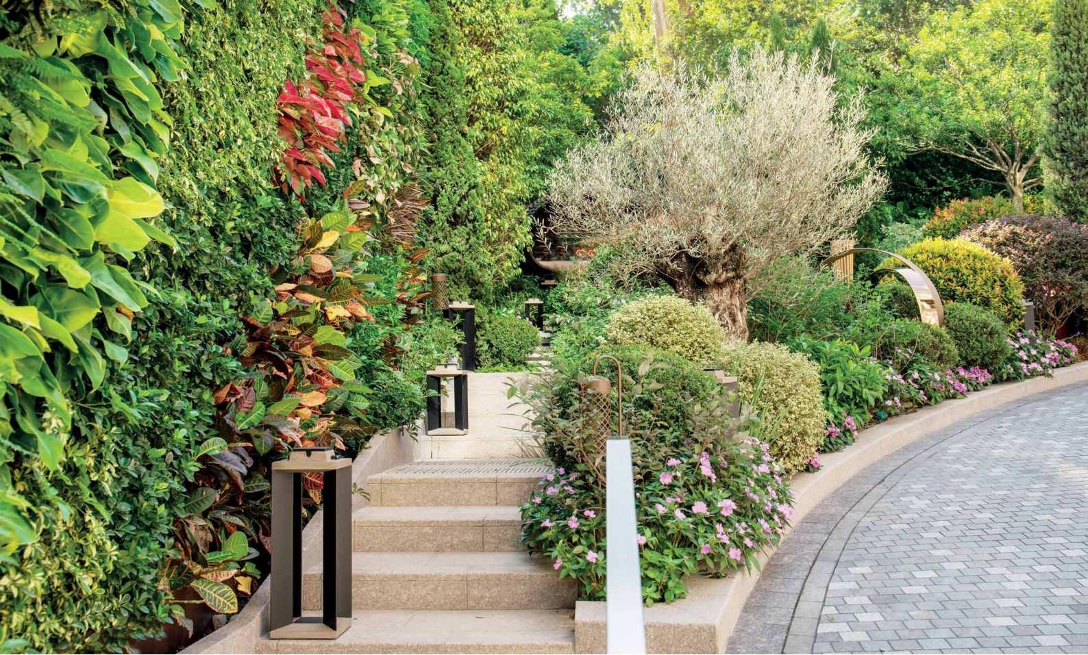
133 Portofino: To enhance water efficiency, the Group collects rainwater for landscape irrigation. 133 Portofino: 集團收集雨水作園景灌溉以提高用水效益。
